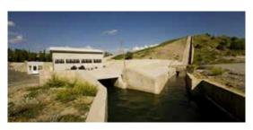
This run-of-river hydropower with reservoir uses three turbines with an annual average of 38 GWh to generate clean energy from the Gölova Dam.
