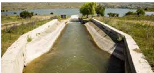
The irrigation canal feeding the Sevindik hydropower station was rehabilitated after damage from landslides and landfalls. As confirmed by the local Water Resource Bureau, there is no negative impact by the hydro plants on water consumption or irrigation.
