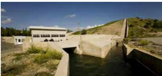
This run-of-river hydropower with reservoir uses three turbines with an annual average of 38 GWh to generate clean energy from the Gölova Dam.
