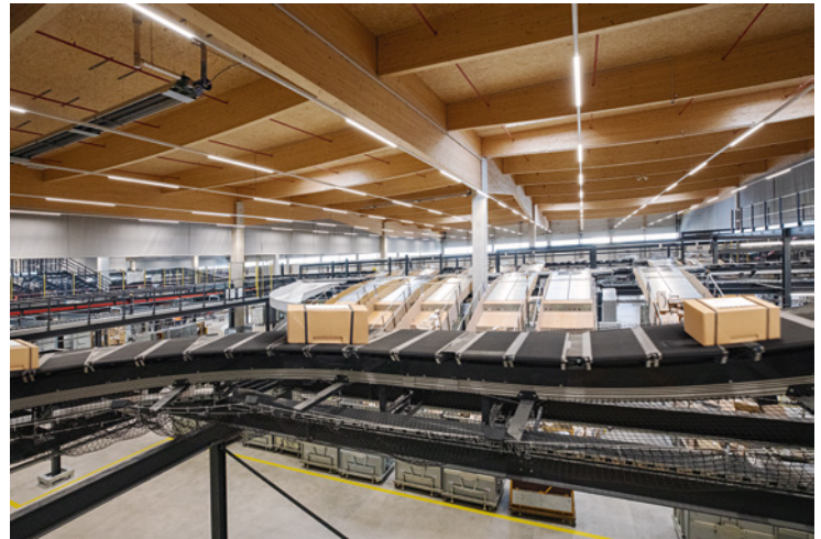
Energy-saving LED technology at our logistics centres
