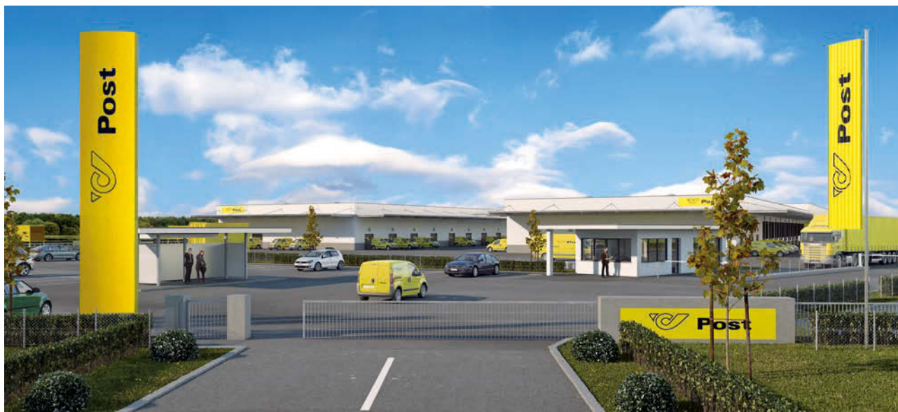
The new Allhaming logistics centre is scheduled to be put into operation in September 2014.
