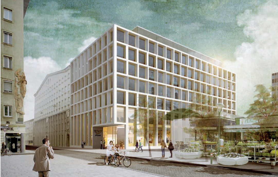
“Post at Rochus”: the new company headquarters of Austrian Post being built in the Vienna-Landstrasse area.
