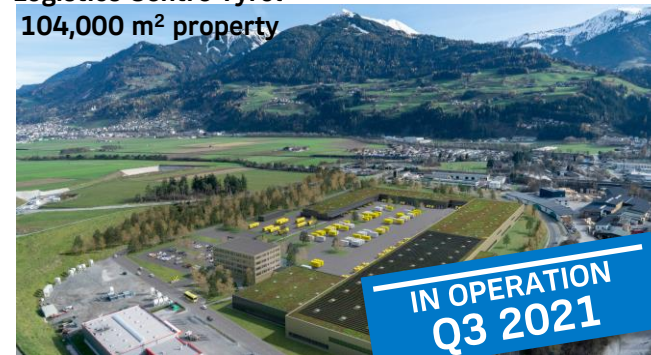
Logistics Centre Upper Austria 126,000 m 2 property
